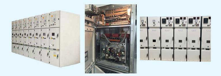
EWC GROUP designs and manufactures Medium Voltage Switchgears (Metal- Clad) type up to 36kV - up to 4000 A - up to 40 kA for 3 sec. with SF6 or vacuum circuit breakers.
